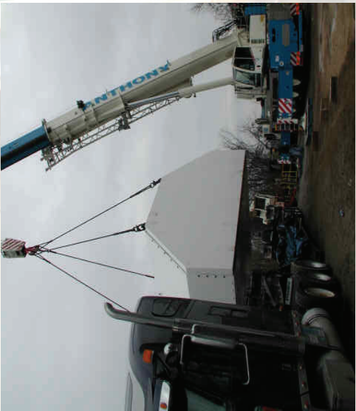
Nuclear Steam Dyer Shipping Container/ Cask For GE Hitachi Nuclear Services
